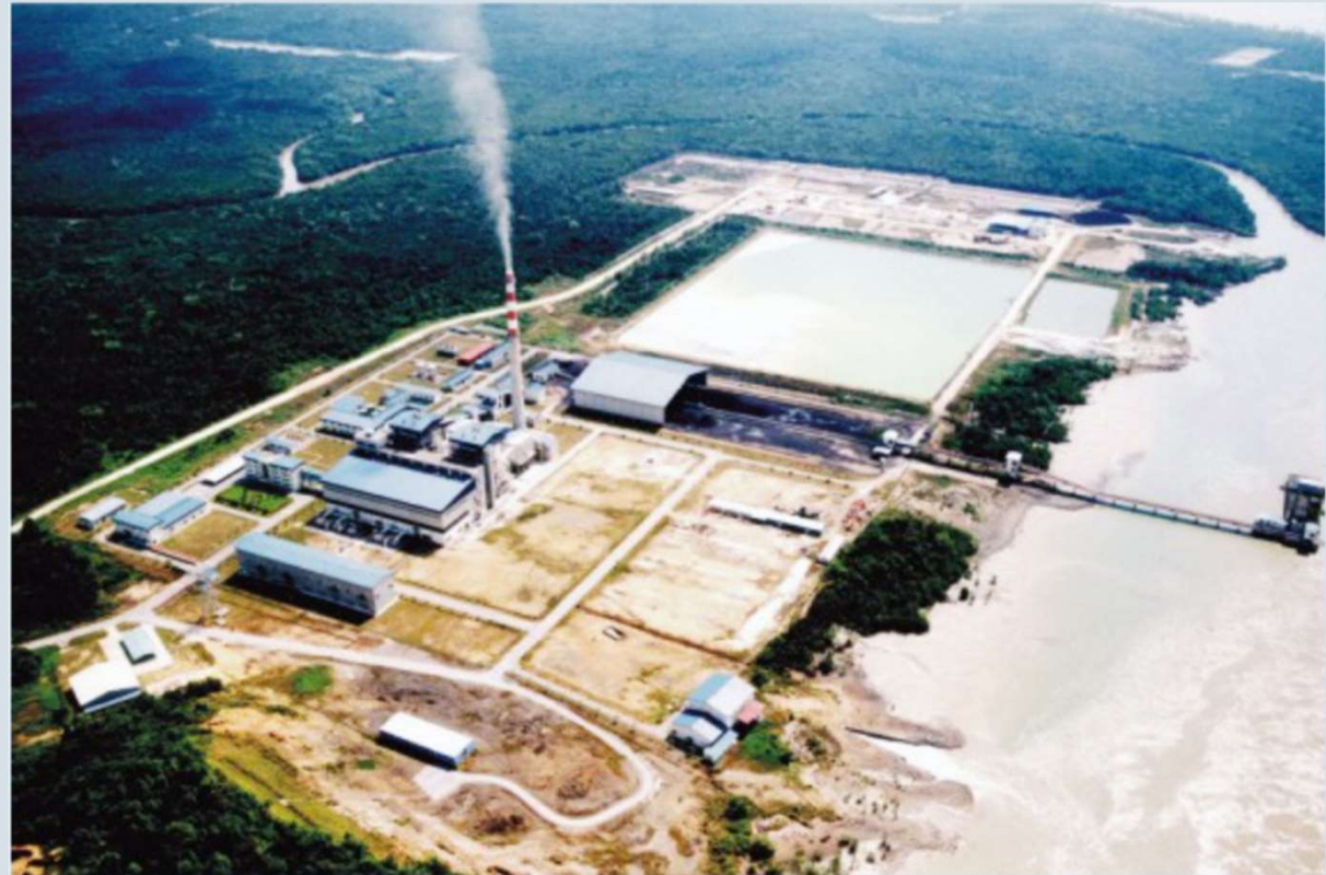
Kuching 2x50MW Thermal Power Plant
