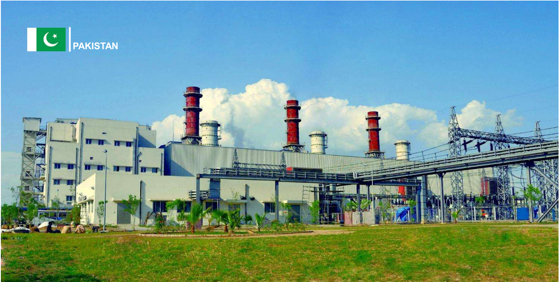
Nadipur 425MW CCPP Project, COD in 2016
