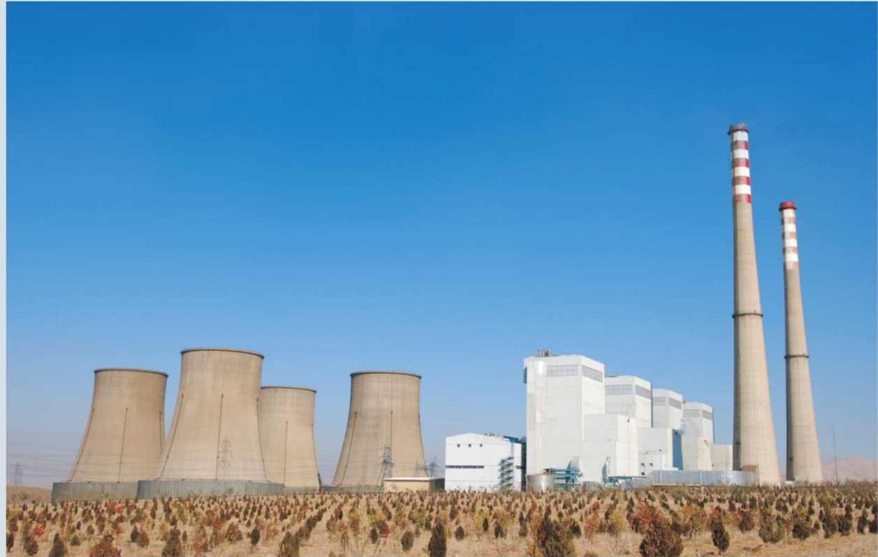
Arak 4x325MW Gas/Oil fired power plant
