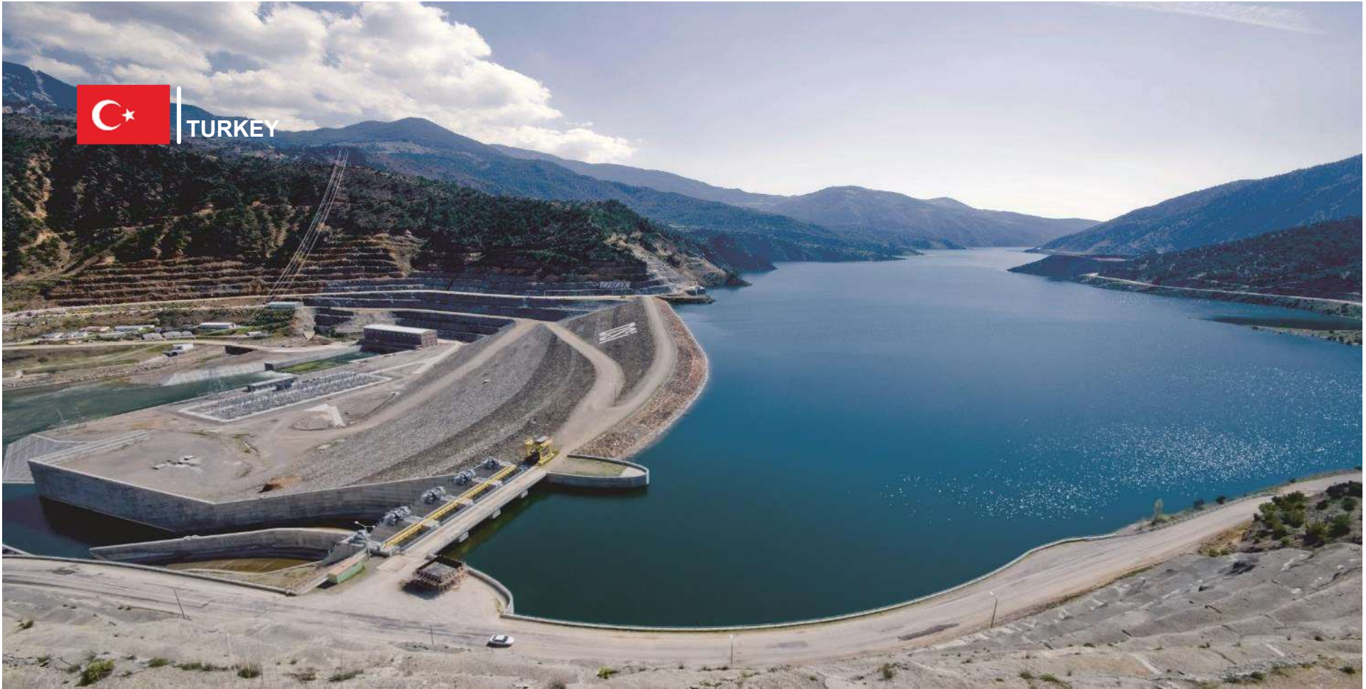
Obruk 4×59MW Hydro Power Project
