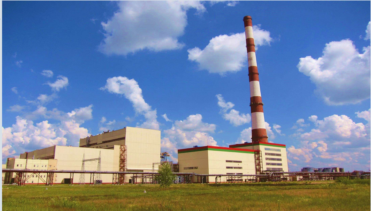
Minsk 400MW CCPP Project, COD in 2012
